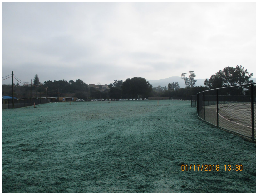
Valley View Elementary School Demolition
