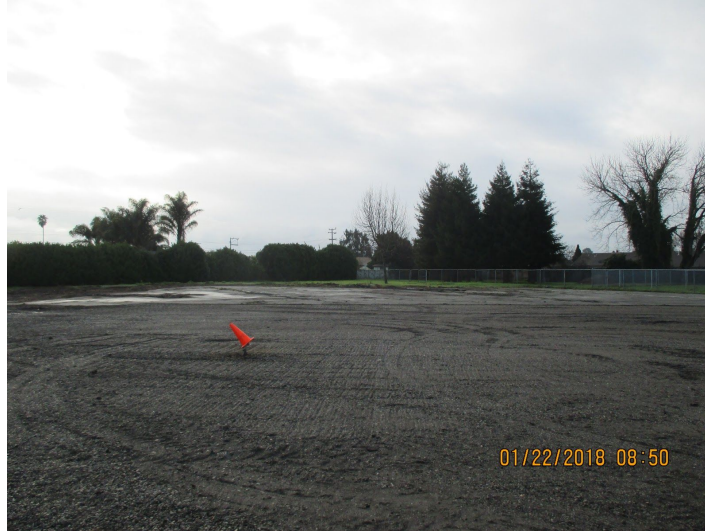
Lake Elementary School Portable Demolition
